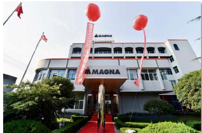
Magna's new engineering center in Shanghai. The center will help deliver the latest mirror and vision systems technologies to Asian markets.
